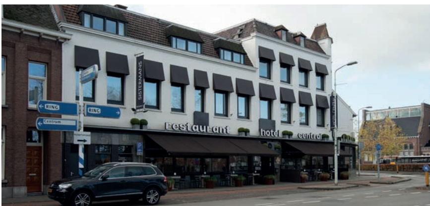
Hotel Central, Stationsplein 7/8/9, 2017.
